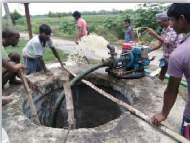
Well cleaning process and Cleaned well with iron net covering and awareness message on the wall
