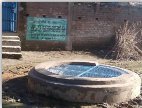
Well cleaning process and Cleaned well with iron net covering and awareness message on the wall
